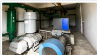
Wastewater Treatment Plant Project Site
